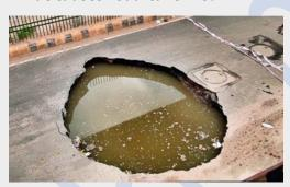
The cave-ins or cavities that look like holes in the ground are a product of the incessant rain. Continuous rain leads to overflowing of drains, which can cause leaks in the pipeline. When a pipeline leaks and water from the pipeline flows into the layers of earth around it, the earth starts to erode and with time, it gets washed away with the water in the pipeline.
